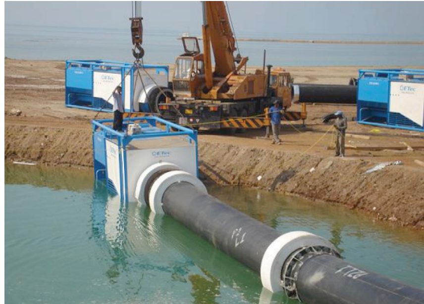
Figure 3. ETEC 48 in floating pumps installation for a project.
